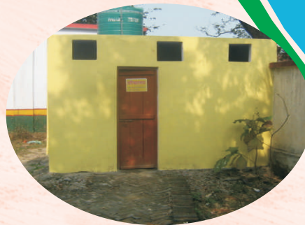
Modern Toilet Construction in 20 School at Varanasi under JOCHNICK Project
